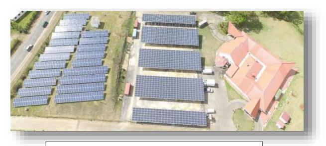
Photo: Aerial view of the 645 kWp solar installation at the Parliament area
