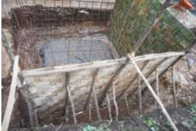
Local labour and local materials were used to assist in construction of the intake tank
