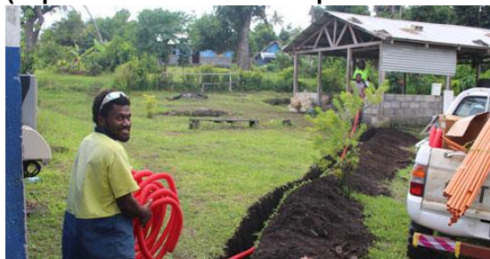
Figure 5: Vate Electrics staff carrying out household service connection process to a household on Tanna Island.
