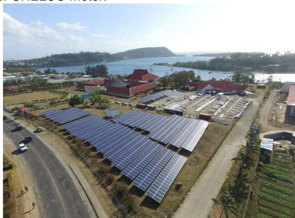
Figure 6: Part of the 767 kW solar plant at the Parliament Park
