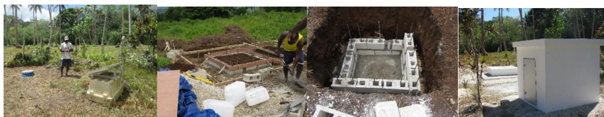
Different stages of station upgrade in SANMA and malekula from the removal of the temporary station to the completion of the permanent monitoirng station shed
