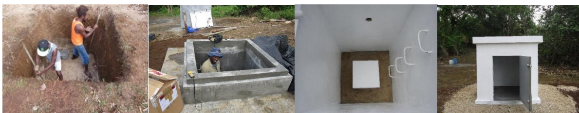
Stages of the shed construction at Ambae at Maewo from the seismic vault digging to the completion of the mini-shed
