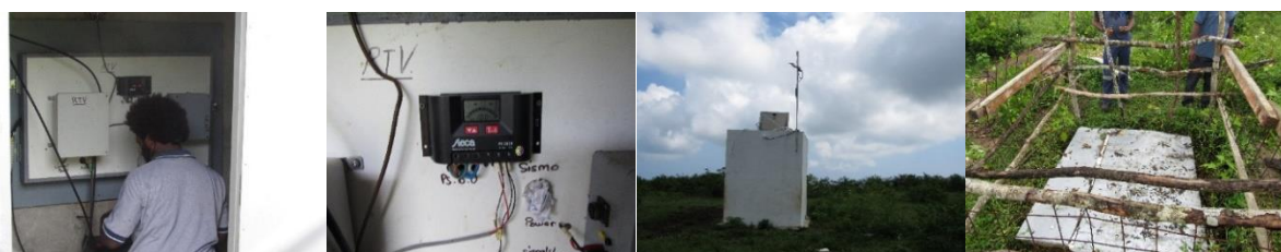
Technician is replacing the regulator at RTV and a temporary fence at MKV station
