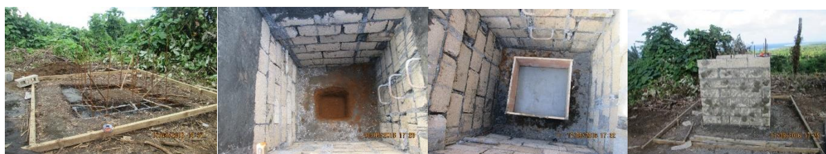
Seismic station shed and slab construction progress at vanua Lava
