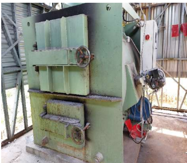
Fig. 4.12 Incinerator at Vila Central Hospital
