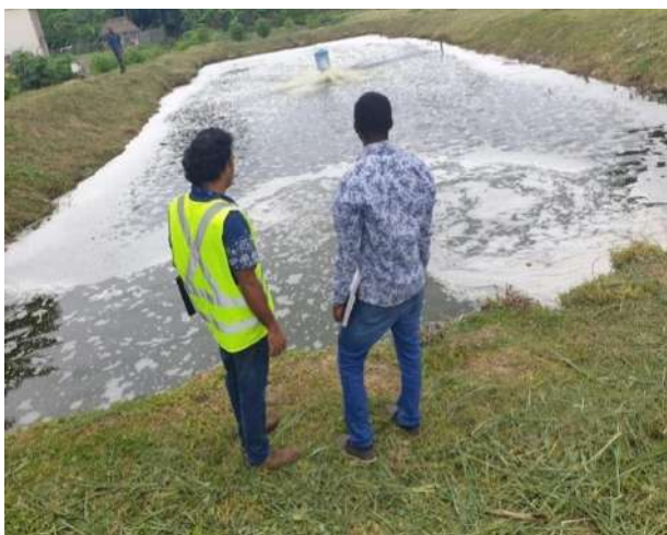
Fig. 4.11 Open aeration system
